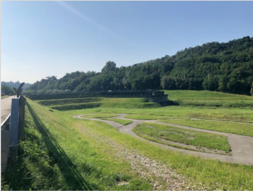
The Gurone on-stream flood detention basin on the Olona river. (image credit: PIANO EMERGENZA DIGA – PED DIGA DI OLONA (VA)..)
