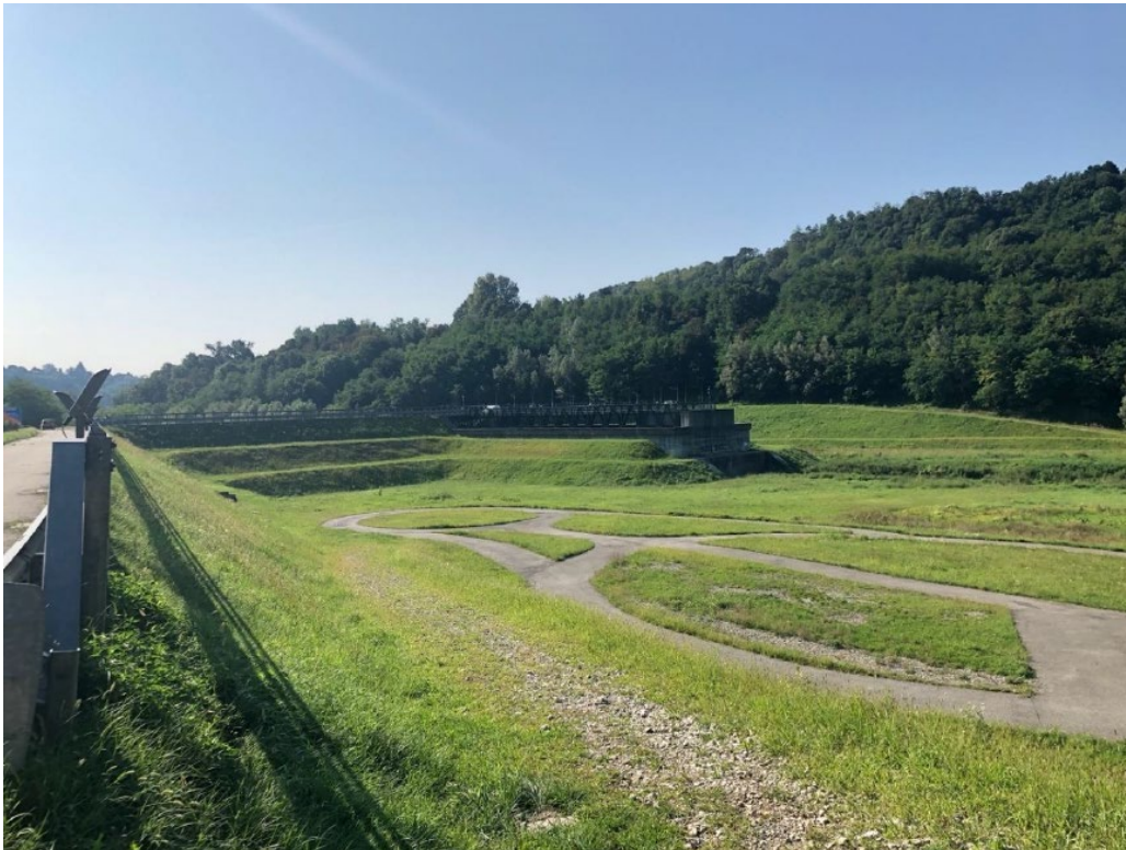
Figure 11.5 The Gurone dam on the Olona river for flood risk mitigation. ( image source: PIANO EMERGENZA DIGA – PED DIGA DI OLONA (VA). )
