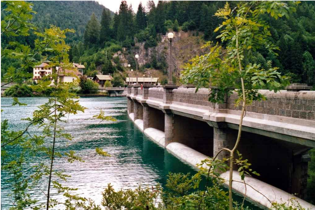
Figure 11.8 Santa Caterina dam, seen from upstream (source: https://progettodighe.it/dighe/santa-caterina/ ).
